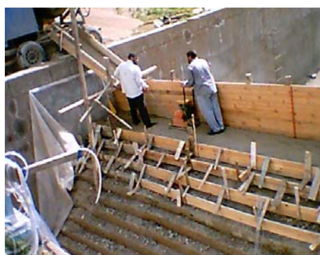
Preparation of protection works
