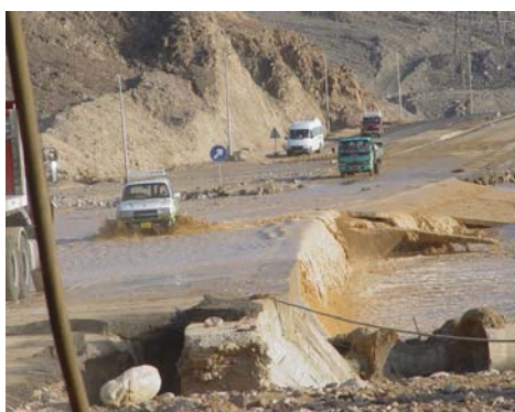
Road in Nuweiba hit by floods
