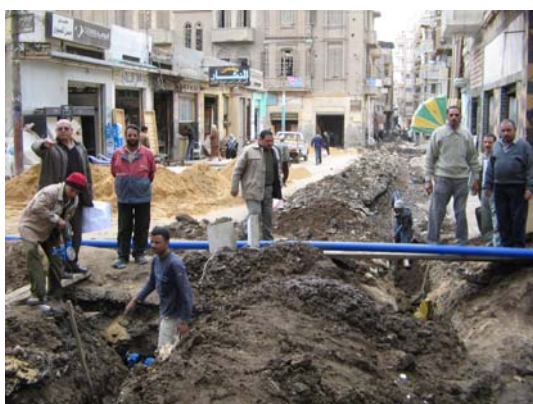
Installation of water pipes in Damanhour
